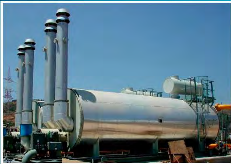
2 FORCED DRAFT WATER BATH HEATERS – 3.900.000 KCAL/h each
