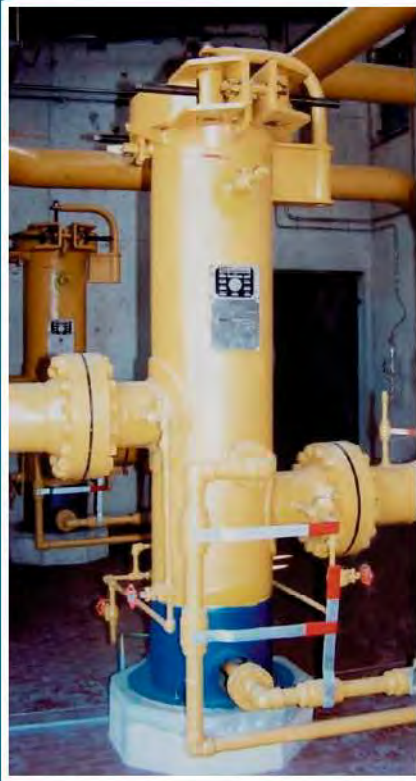
2 GAS FILTERS FCV TYPE - 20" # 600
