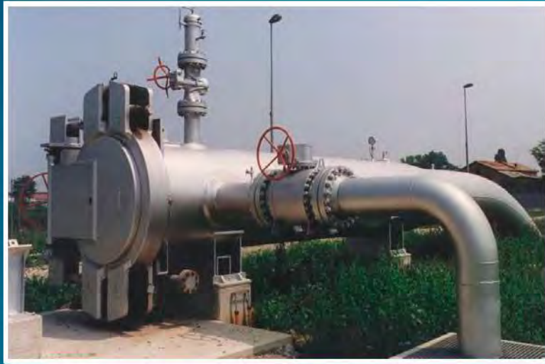
BIDIRECTIONAL TRAP 48" x 56" # 600
