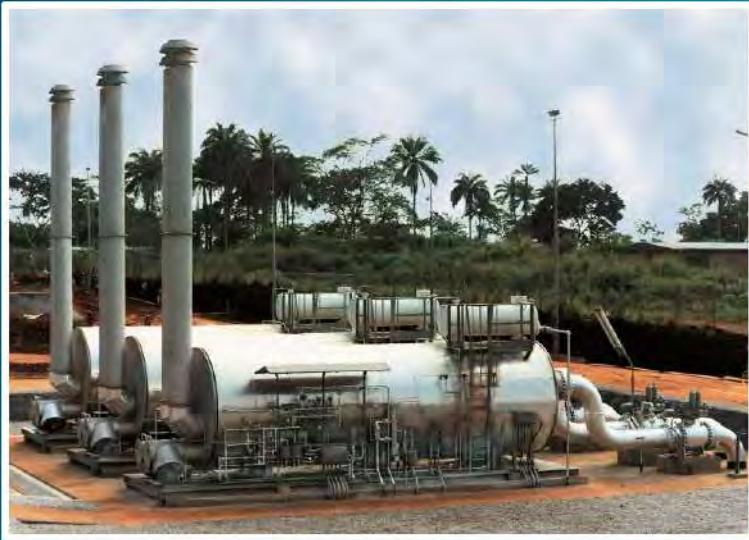
3 NATURAL DRAFT WATER BATH HEATERS – 2.000.000 KCAL/h each
