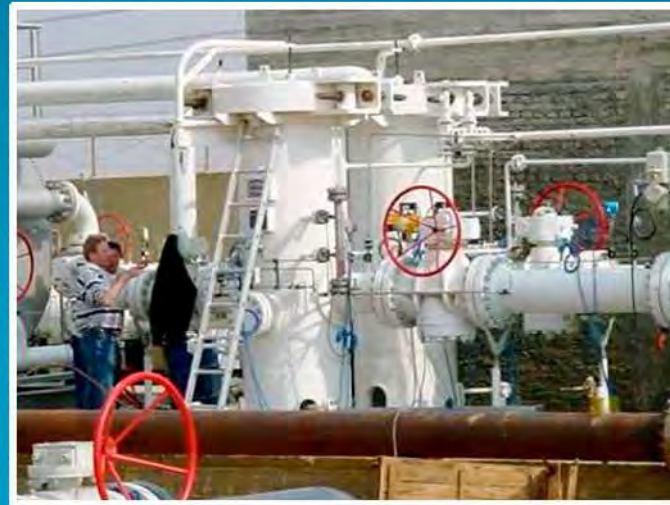
2 GAS FILTERS FCV TYPE - 34" # 600
