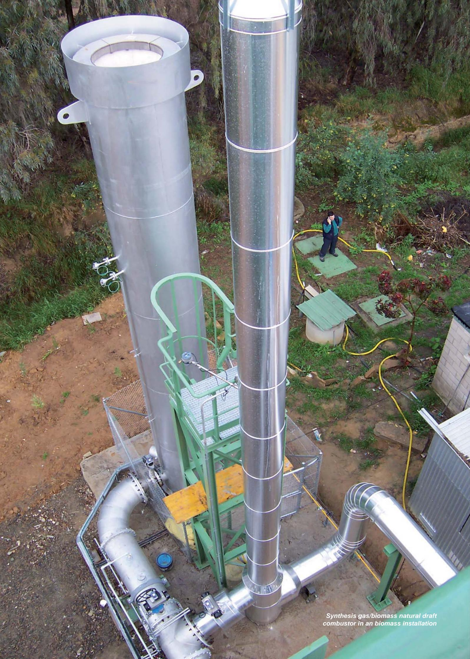
*Synthesis gas/biomass natural draft combustor in an biomass installation*
